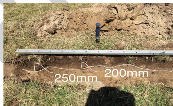
Figure 9 "Trevista" Looking SE. This is a cross-section of trial plot A&B. Note the valleys created by the slippers and the humps of the compacted soils. Average depth about 150mm.
