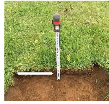
Figure 23 The white line in this photograph delineates the root layer from the clearly defined compacted zone. The root depth is approximately 40mm.
